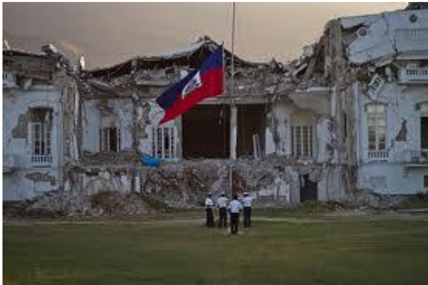
Figure 7 The Presidential Palace after the earthquake - The Guardian
