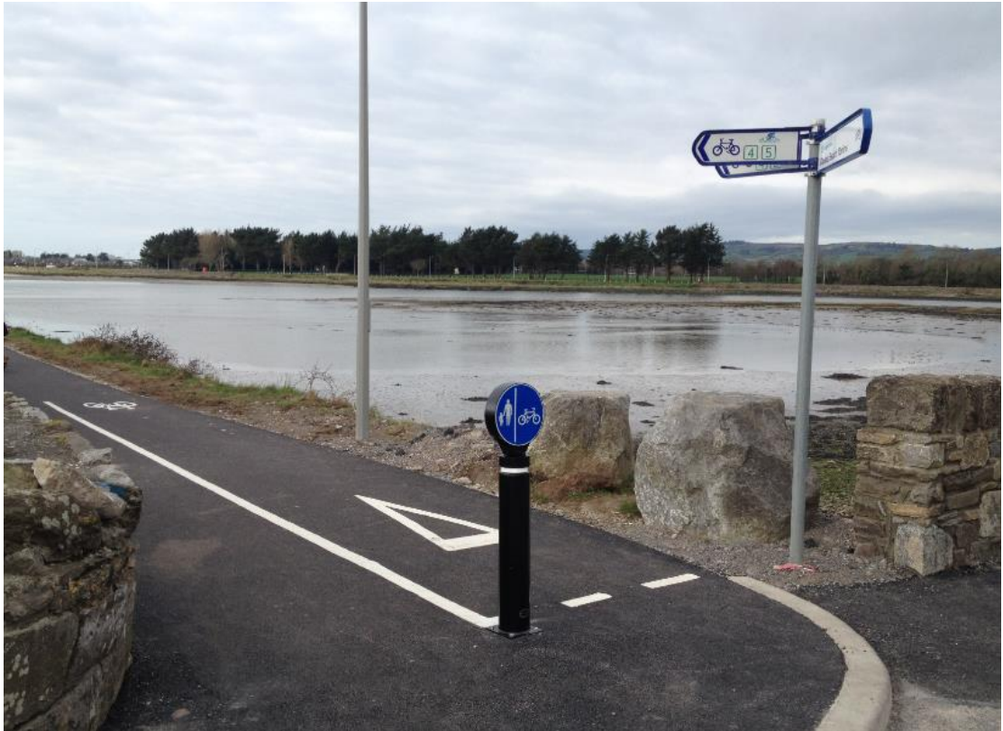
Converted railway line for active travel near schools in Duckspool area in intervention town 2
