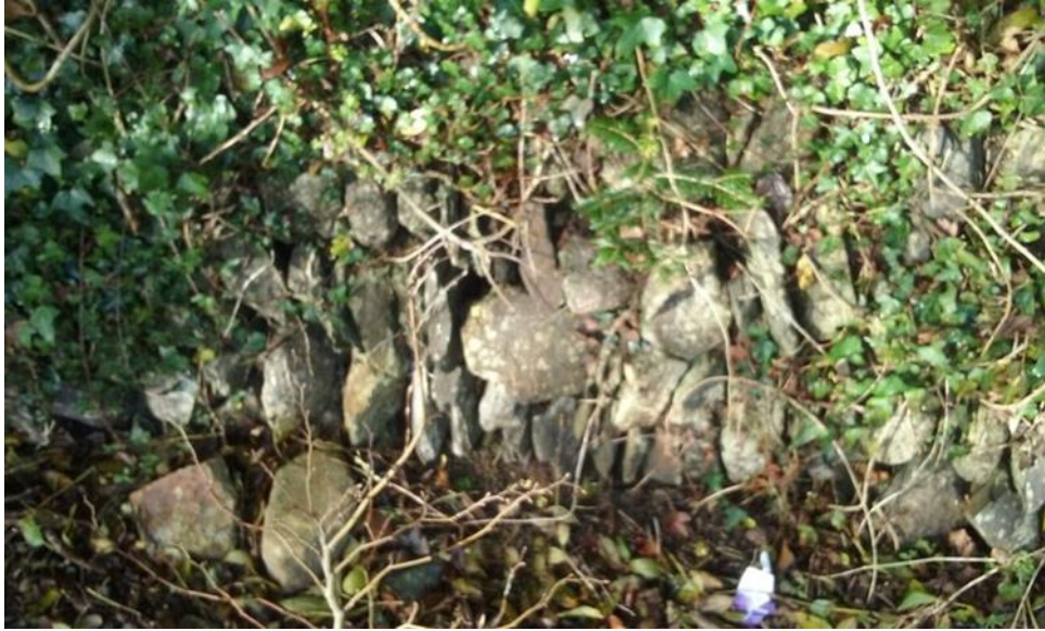
Figure 7.15 Dry stone wall
