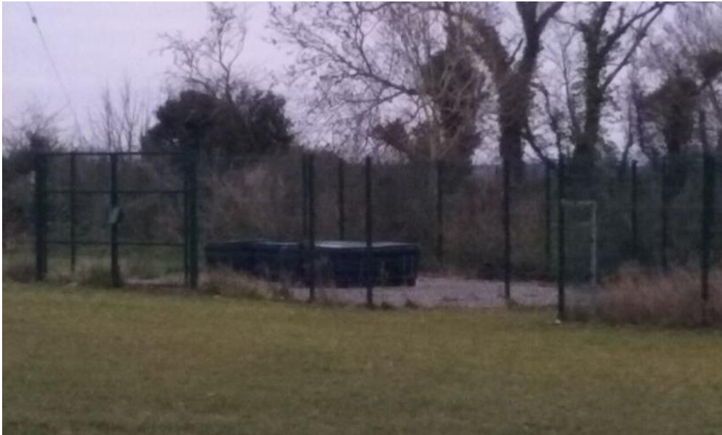
Figure 7.5 Water treatment system at the back of the school.
